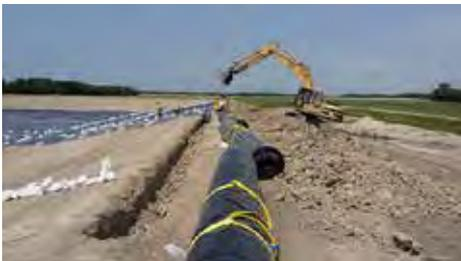
at a new waste management facility in Port Hope where they installed over 900,000m<sup>2</sup> of HDPE geomembrane, geotextile and geosynthetic clay liner (GCL) to three radioactive waste cells.
