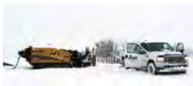
Installing fiber in the middle of winter. Photo courtesy of Accurate HD. Member profile, page 10.
